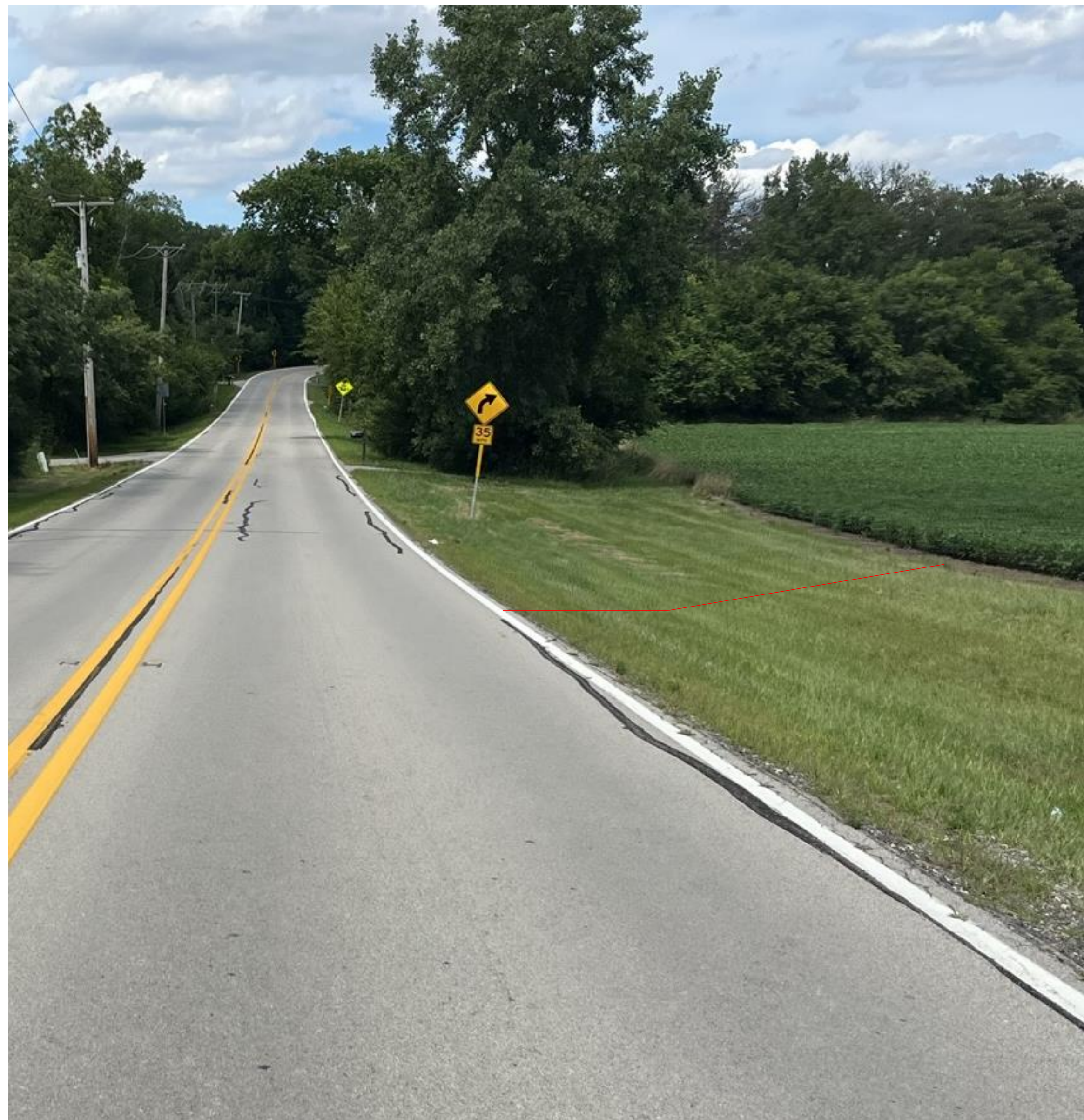
Shallow ditch, no capacity
